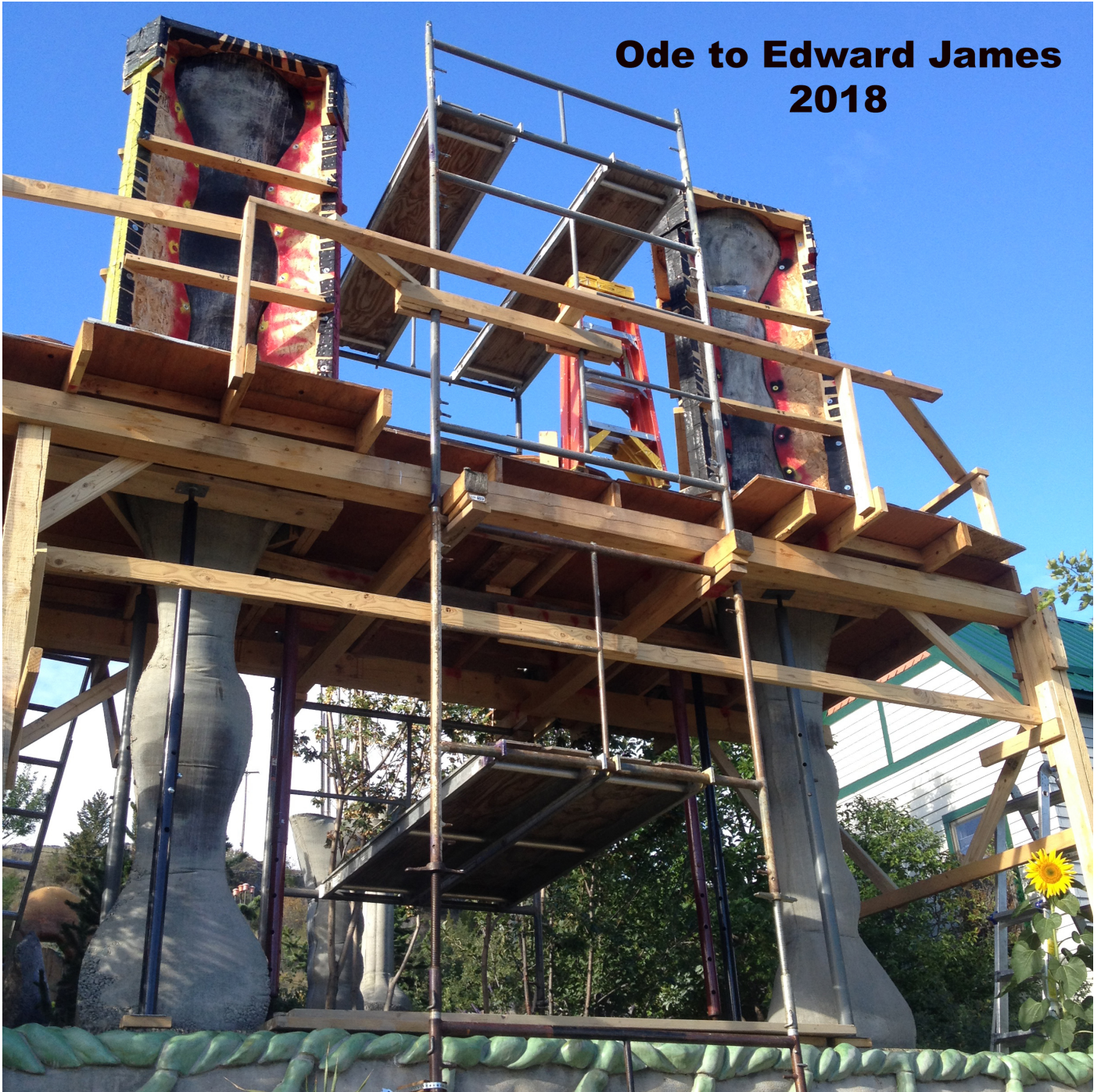
Clawson_07 Ode to Edward James – 2018 – The sculpture under construction showing the relationship of the poured columns to the already poured columns. This sculpture was under construction for three years.
